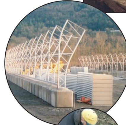
**Diamond Shelter** Welded Truss frames are constructed of hollow structural tube with yield and tensile strengths that allow them to withstand heavier stress loads. All frames are engineered to meet the requirements of the National Building Code.
