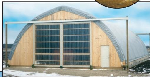
Double Sliding Doors covered with translucent panels create an appealing finish to this 40' x 72' **Diamond Shelter**.
