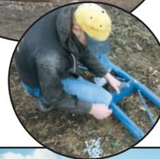
◀ All rafters and cross bracing have easy to assemble bolt together joints.
